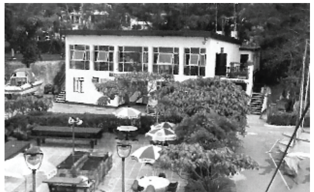
HHYC clubhouse and BBQ garden upgrade 1984
